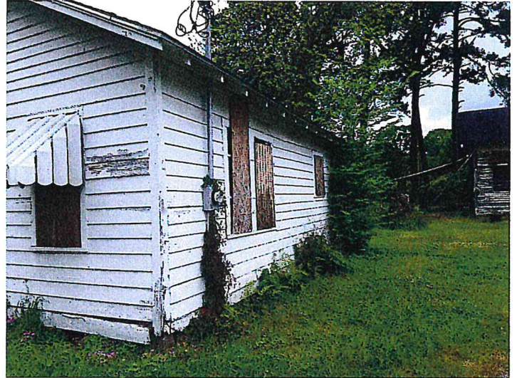
4/19/2016 EXTERIOR SIDE D - 513 C NE EVANGELINE THRUWAY Pic (19).jpg
