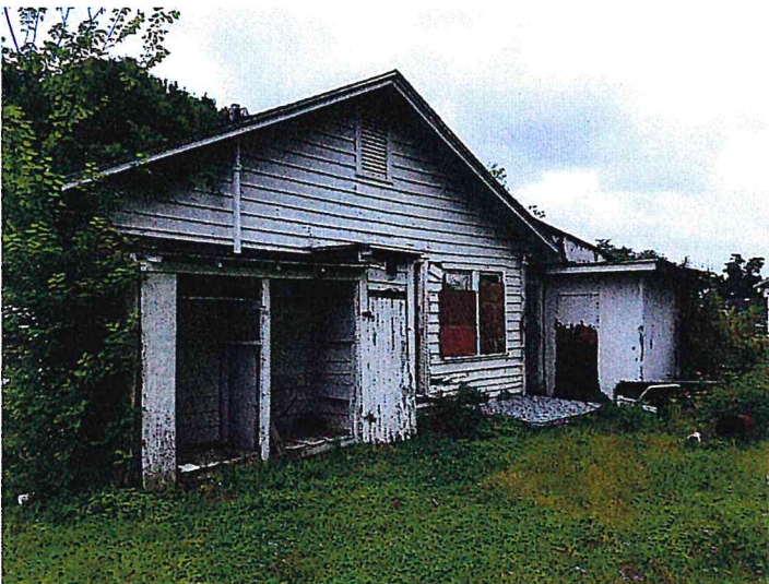
4/19/2016 EXTERIOR SIDE C - 513 C NE EVANGELINE THRUWAY Pic (20).jpg
