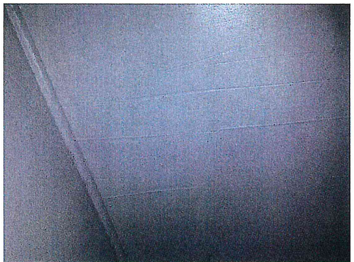
4/19/2016 SAMPLES S13 & S14 - GYPSUM BOARD CEILING Pic (29).jpg
