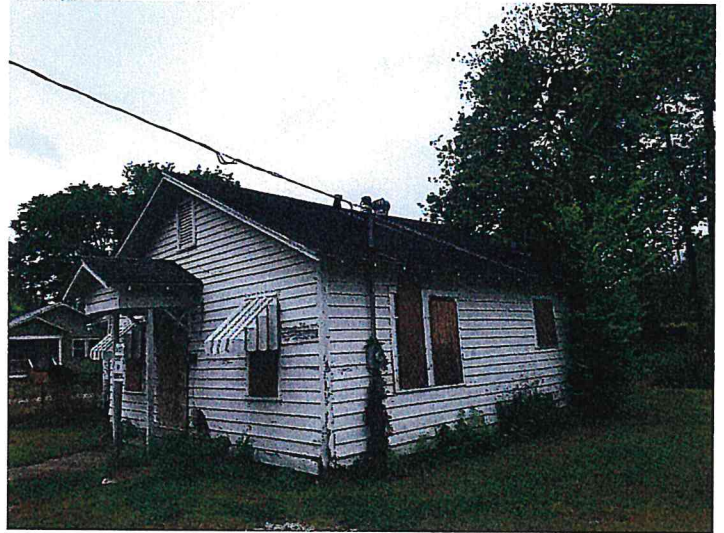
4/19/2016 SAMPLES S51 & S52 - SHINGLE ROOF & FELT MTRL Pic (31).jpg
