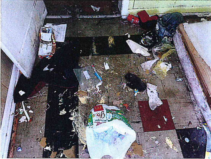
4/19/2016 513 C - INTERIOR Pic (26).jpg
